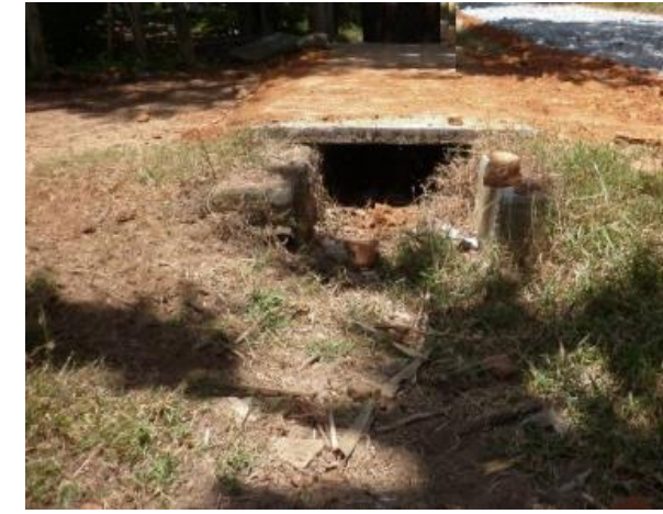
Fig.3.3e: Cross drainage culvert with inadequate capacity/not well maintained and unlined open channel used to convey accumulated stormwater to downstream floodplain
