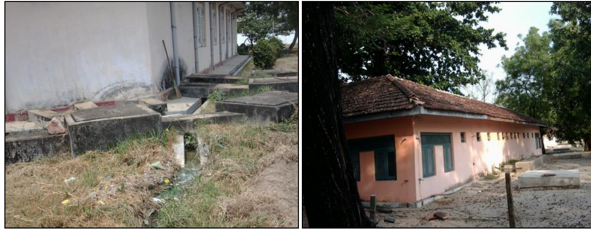
Fig. 3.3b: Gutter drains not connected to main drainage lines with open ditches with inadequate capacity (Left) and Broken roof gutters (Right)
