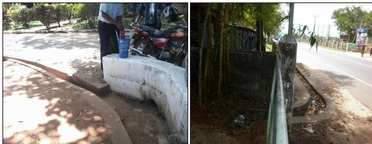
Fig. 3.3d: Silted/partially blocked cross drainage culvert (Left) and Blocked roadside (toe) drainage line (Right)
