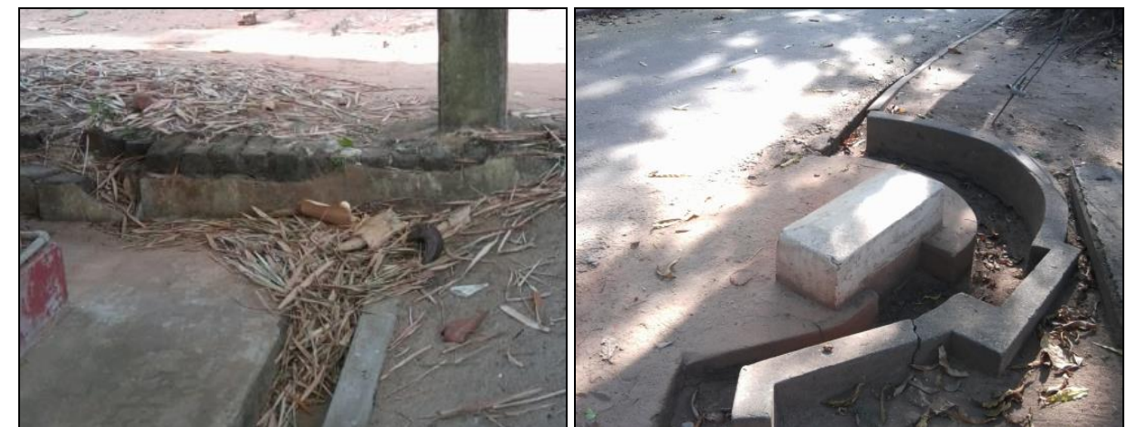
Fig. 3.3a: Blocked gutter drain (Left) and silted drain with blocked/closed culvert (Right)
