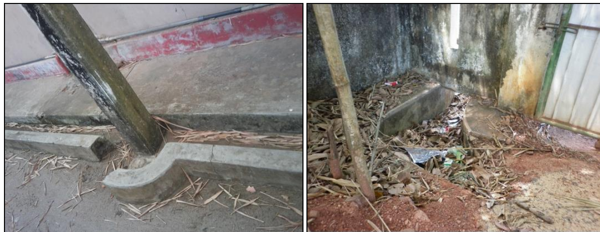
Fig. 3.3c: Blocked, discontinued and leaking gutter drain (Left) and Blocked/silted main drains (Right)
